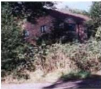
A recently built, traditional design cottage. Retention of the mature hedge is good practice
