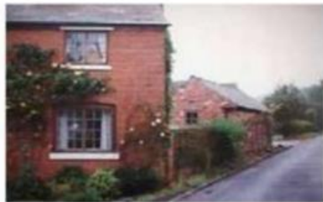
A recently-built garage, making good use of reclaimed bricks, slate roof and wooden window frames, to blend with the original cottage
